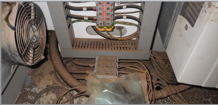
▲ OMAX waterjet cutter control cabinet before decontamination
