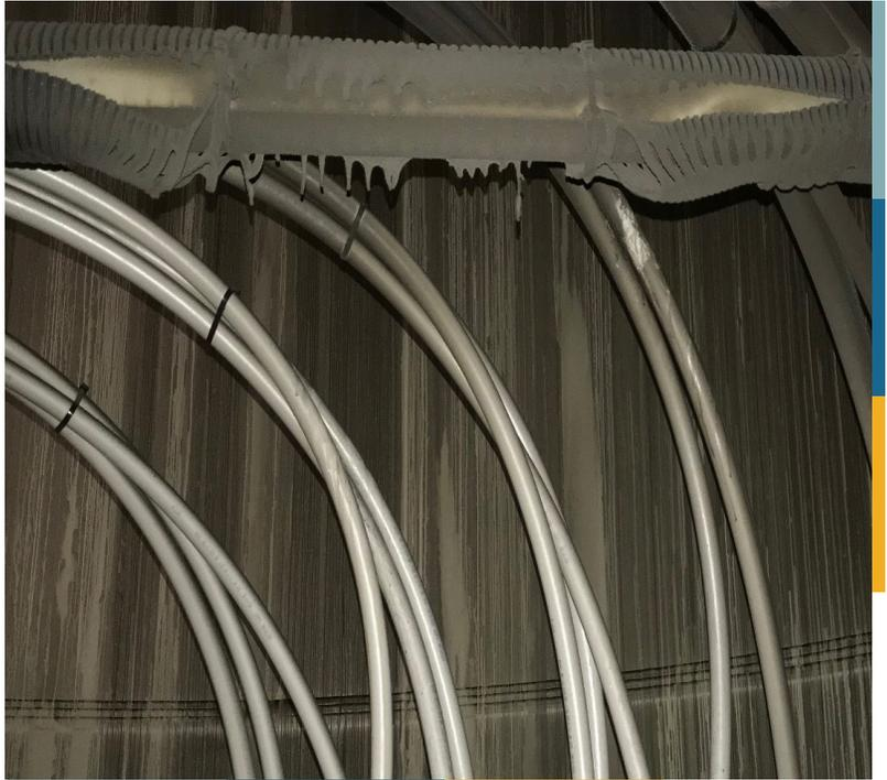
*The melted PVC, at the top of the photo above, is a clear warning. PVC releases large amounts of hydrochloric acid in the combustion process and corrodes metal surfaces.*
