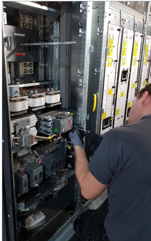
▲ The container and switchboards being disassembled
