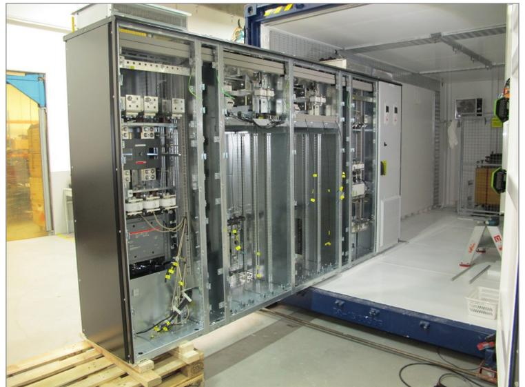
▲ Reassembly of electrical switchboards and container
